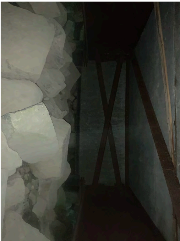
Right Bank Abutment when facing downstream
