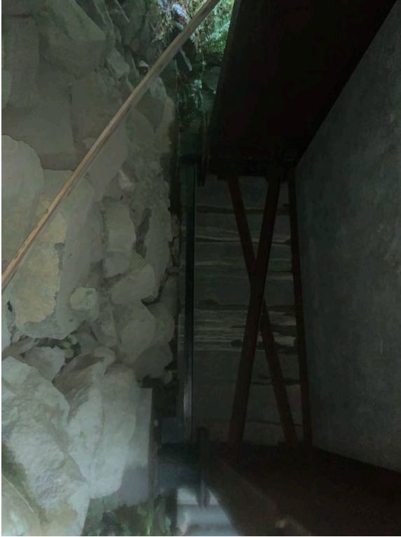
Left Bank Abutment when facing downstream
