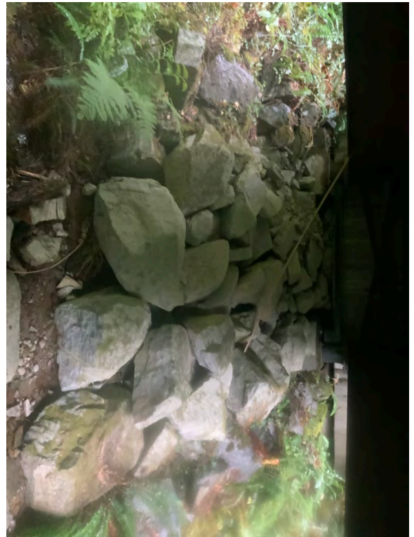
Left Bank Abutment when facing downstream
